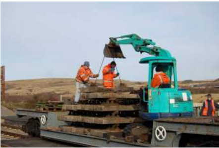
Loading sleepers at Furnace Sidings with the mini digger
