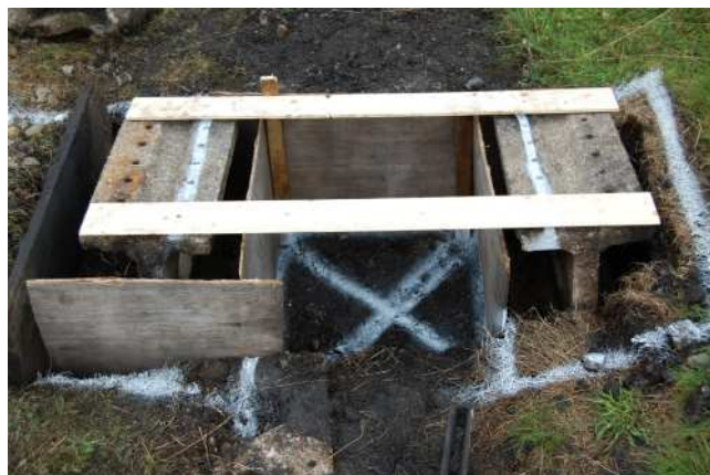
Above—the new settings for the ground frame prior to the pouring of the concrete. Andy May
